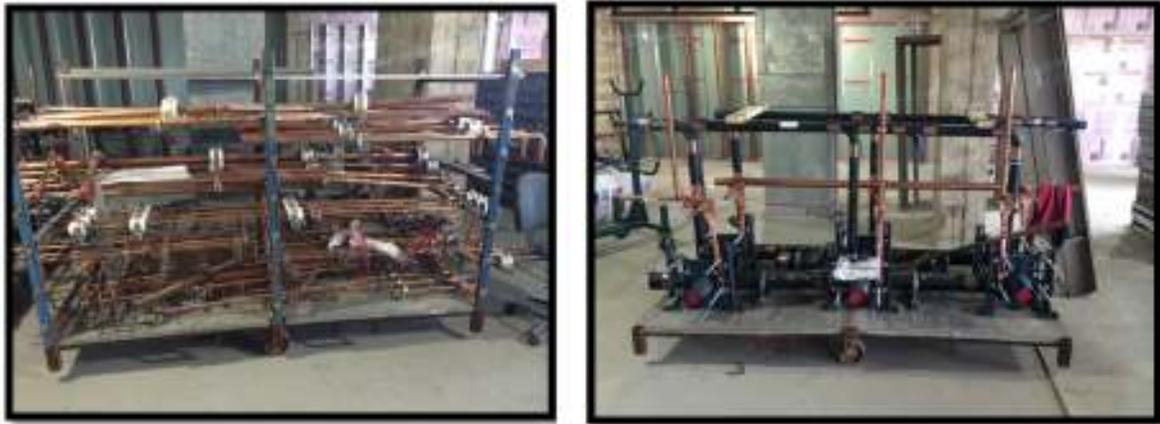
These racks allow workers to easily transport large amounts of preassembled piping systems from the trailers they are brought to site on and then rolled onto a material hoist or service elevator to bring them to the proper floor for installation. Once at their proper location the pieces are taken off the rack and lifted into place where the final connections are to be made.
